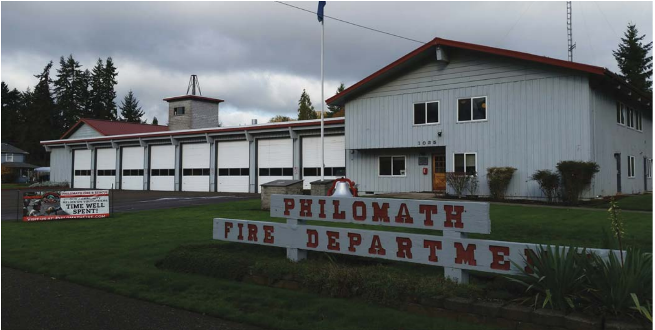
VIEW OF FIRE STATION 201 (FROM SOUTHEAST ON MAIN STREET)
